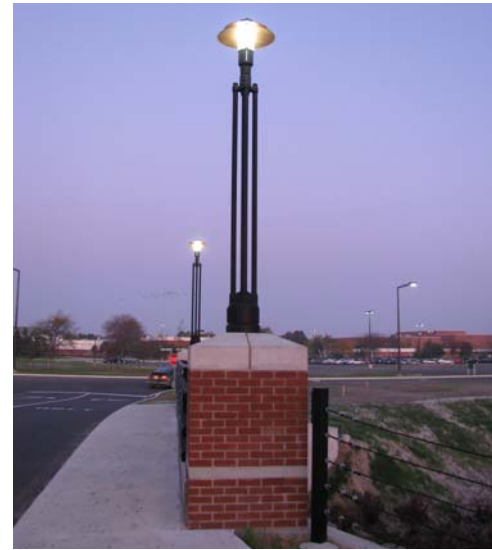
(Above) Examples of LED lighting at Delta College
